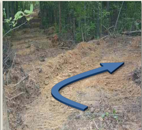
Turnout used in conjunction with a waterbar to disperse runoff water
